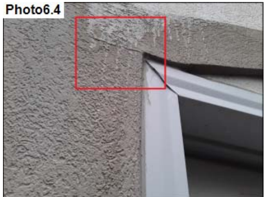
Compression Crack
