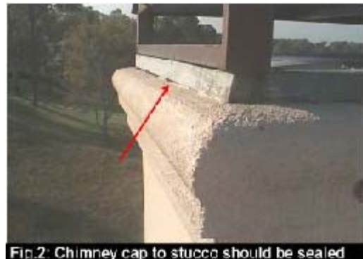
Fig.2: Chimney cap to stucco should be sealed
