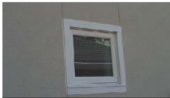
Figure 2: Typical outset window detail (sealed)
