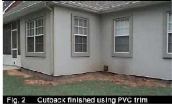
Fig. 2 Cutback finished using PVC trim
