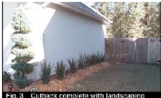
Fig. 3 Cutback complete with landscaping
