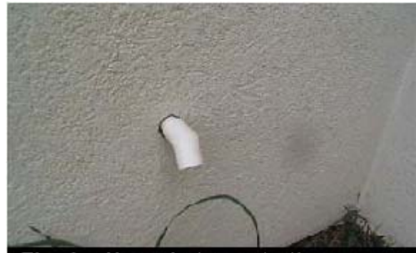
Fig. 1 Unsealed penetration
