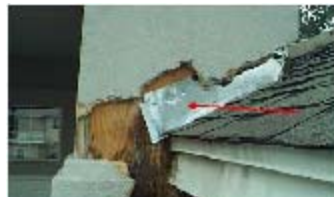
Figure 3: Failed flashing
