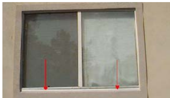
Fig. 4: Window sealed using barker rod at bottom
