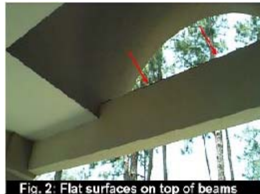
Fig. 2: Flat surfaces on top of beams
