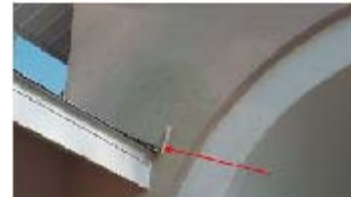
Fig 4: Proper repair kickout installation
