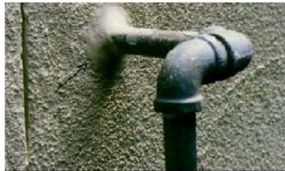
Fig. 2 Sealed pipe penetration
