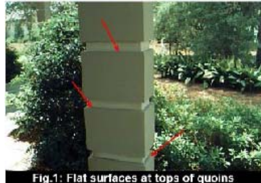
Fig. 1: Flat surfaces at tops of quoins
