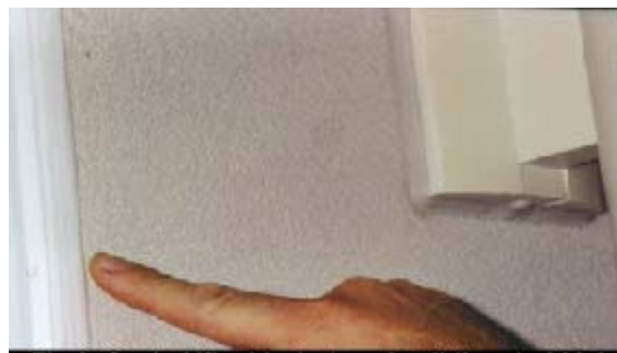
Fig. 3: Sealed 'flush' window detail (band-aid joint)
