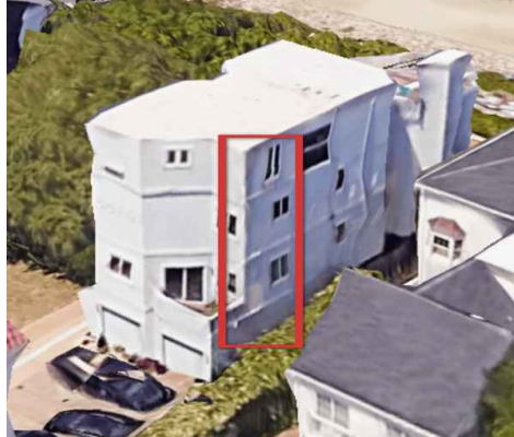
Bulging wall due to moisture intrusion
