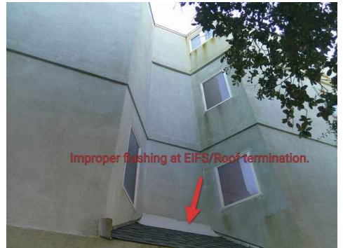
Improper Flashing
